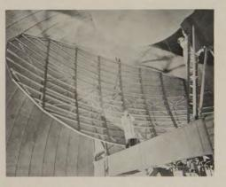
SEARCH RADAR produced by General Electric detects air targets at greater ranges and higher altitudes than present detection systems. This FPS-7 system determines height, range and azimuth simultaneously.
